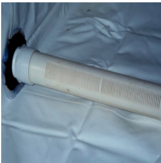
Picture 5. Bed with liner and well screen
