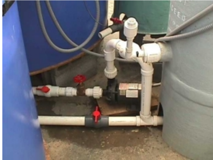
Picture 1 – Installation of pump between fish tanks and beadfilter.
